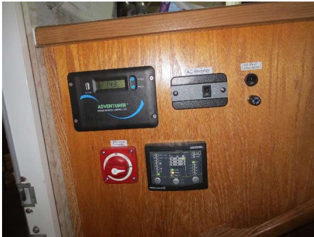
Shore and Solar charging control panels Solar shut off switch and hot water recirculatory switch
