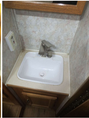
Upgraded sink and faucet
